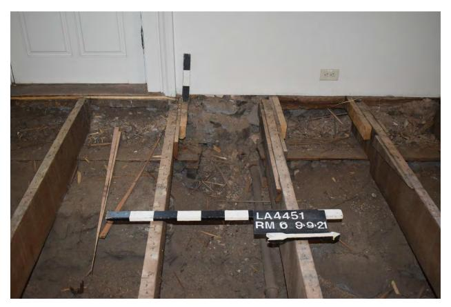
Figure 31. Typical joist-wall junction along the west (Lincoln Avenue) wall of Room 6.
