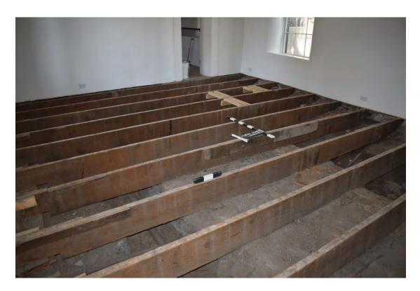
Figure 27. Overview of Room 6 from the southwest room corner. Note the blocking reinforcements near the door to Room 19.
