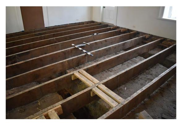
Figure 28. Overview of Room 6 from the northeast room corner. Note that the joist ends are supported by a constructed shelf adjacent to the Lincoln Avenue wall foundation.
