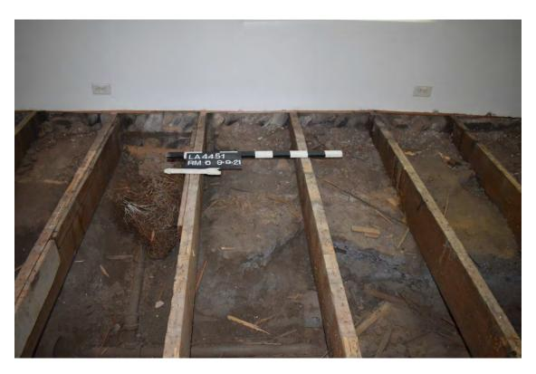
Figure 32. Typical joist-wall junction along the east (courtyard) wall of Room 6. Note the greater depth of sediment that has accumulated against the joist surfaces and that will need to be removed.
