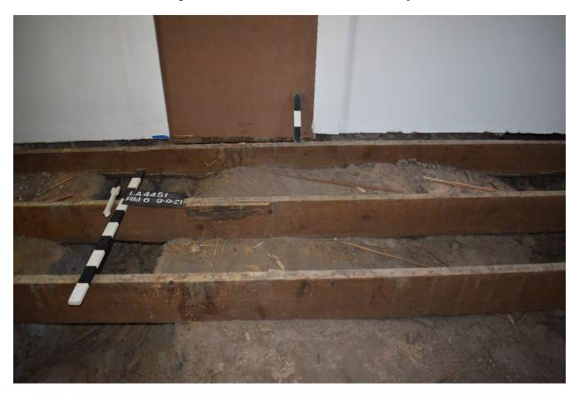
Figure 36. The southern three joists within Room 6. The southernmost joist may require complete replacement due to condition issues.
