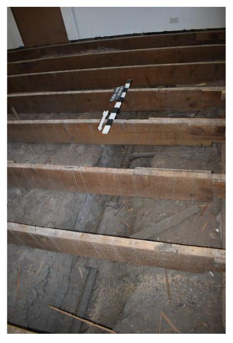
Figure 30. Detail of the eastern the sub-joist trench and its gas line. Note the larger diameter pipe sleeve in the main trench.
