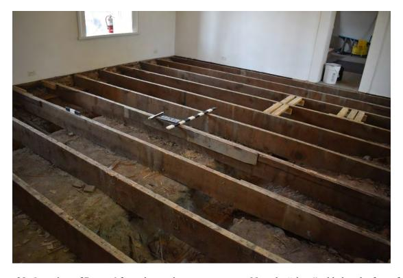
Figure 28. Overview of Room 6 from the southeast room corner. Note the "sister" added to the face of the joist under the metric scale.
